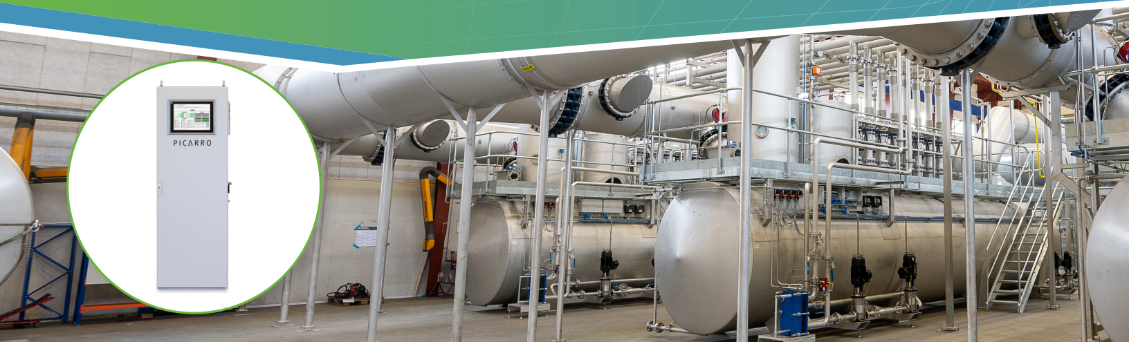
Figure 1: LESNI EO Catalytic Abatement Plant (EO CAP), with Picarro Continuous Emissions Monitoring System (CEMS) inset.
