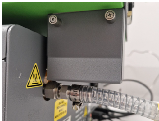
Figure 25 - Vaporizer to Analyzer Installation Complete
