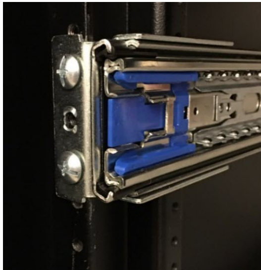
Figure 15 - Outer Rail Mounted to Rack
